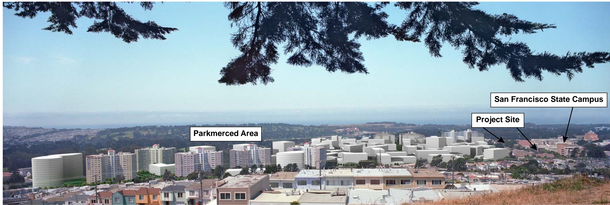
Future Conditions with Buildout of the Parkmerced Project
